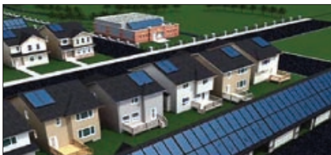
EnerWorks panels installed at a solar community in Okotoks, Alberta, the largest installation of solar thermal technology in Canada
